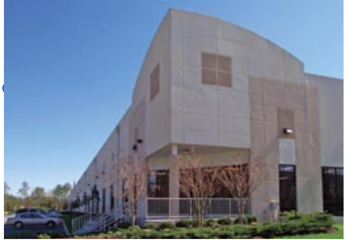
Rivers Bend Warehouse makes a dramatic statement for any business leasing space here.
